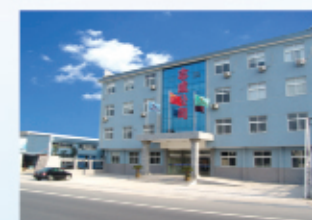
南厂区 South Plant
